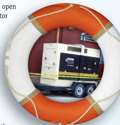
Emergency generator powering an entire business, allowing normal operations weeks before utility power restored.
